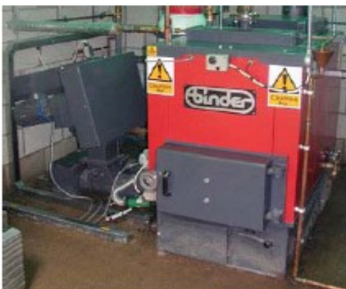
Figure 6. Binder (50kW) wood chip boiler meets 50% of large educational centre's hot water
