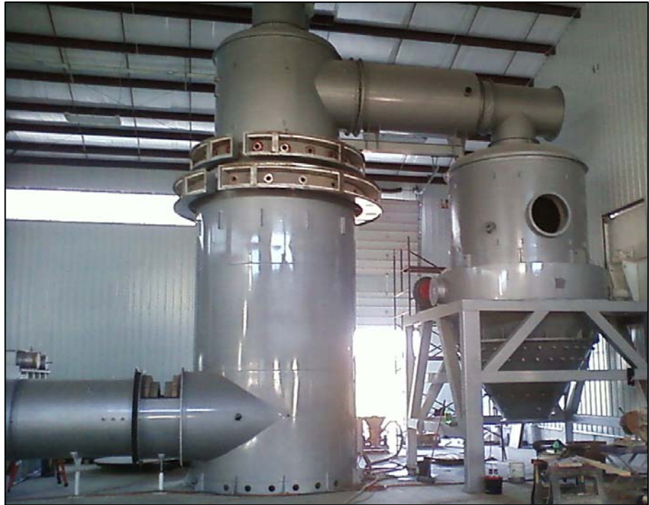
Construction of an HTI Fixed Cell Gasifier and Oxidizer
