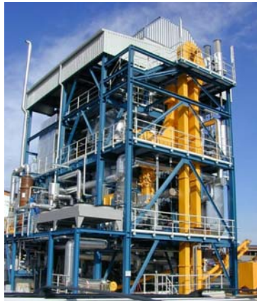
Figure 16. Picture of the biomass CFB steam gasification process in Güssing (A)
